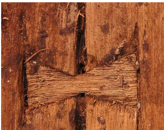
Fig. 7. Coffin tenon construction.
