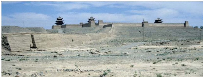
The Ming Fortress at Jiayuguan, blocking passage through the Hexi Corridor.
