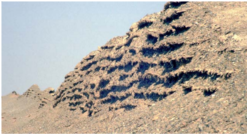
Fig. 3. The Han wall at Yumenguan, showing stamped earth construction.
