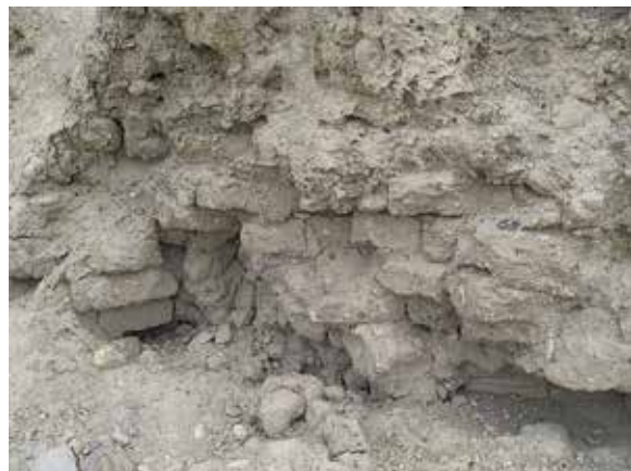
Fig. 9. Detail of mud bricks at Arzun fort.
