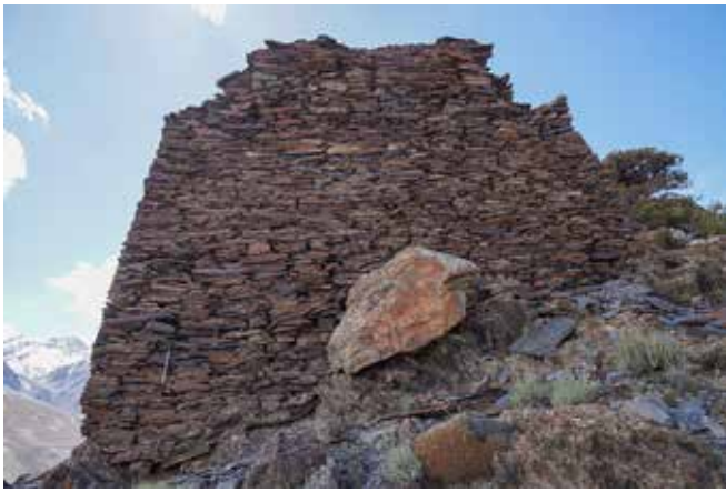
Fig. 11. Eastern wall of the Zangkuk watchtower.
