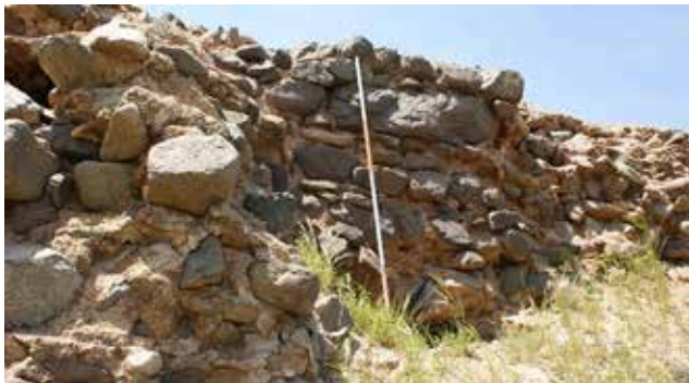
Fig. 14. Masonry of the fortress walls.
