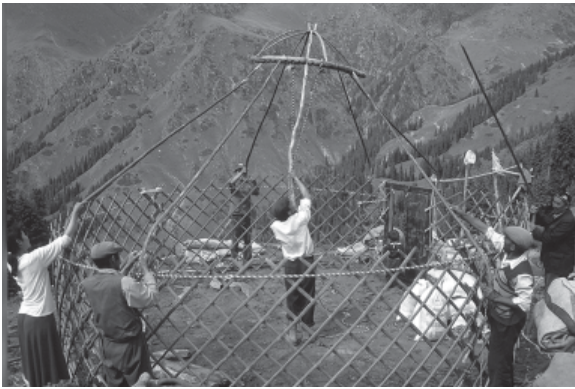
Erecting the frame of the yurt
